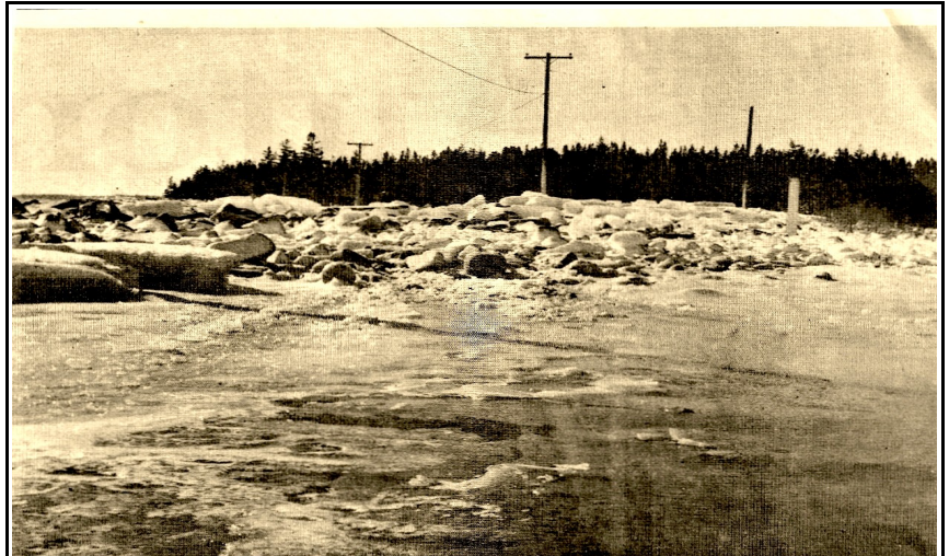
Stormy Feb 7, 1978. Started abt. 11:00 am - right before Boston hit us hard. Seawall Roadblock Last week's storm piled chunks of sea ice 12 to 14 inches thick over Rte. 102A at Seawall. Behind the ice pile, rocks and ice wedged out the road and left it strewn with debris and debris the length of the seawall. No one in the area can remember so much storm damage to the road; it was washed out in the 1930's but not as badly. Photo by LaRue Spiker
